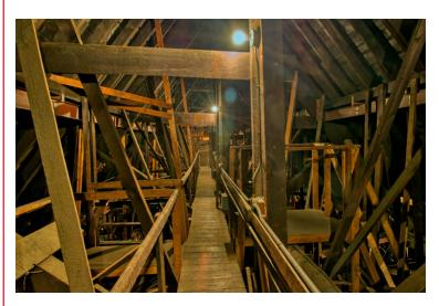
The space above the church ceiling has been modified by changes in the heating/cooling systems and by the impressive addition of iron reinforcing beams in the 1980's. Heroic efforts also prevented a fire from spreading over the chapel at one point; we did not explore in that direction but all of the largely wooden bracing seemed fine from the main walkway.
